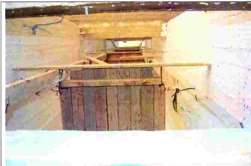
Phase n.2 – Building n. 1 – Scaffolding in the elevators shafts
